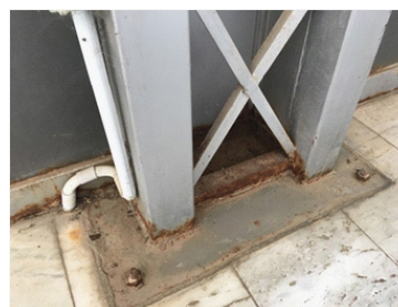
Fig. 8: The building pillars with corrosion at the bases
