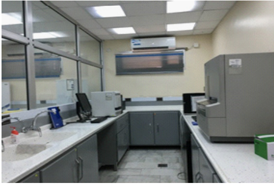
Fig. 11: The new sinks (left hand side) are made of chemical-proof materials
