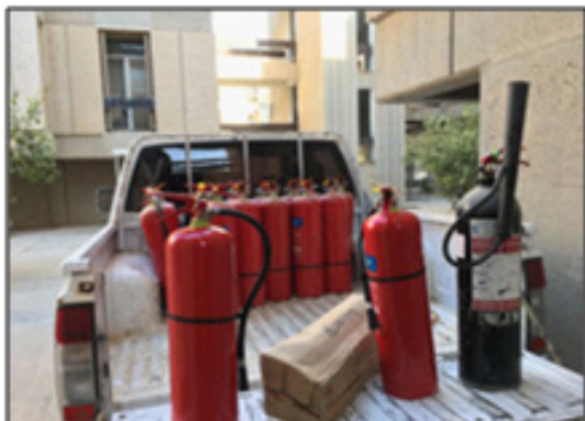
Picture 4: Fire extinguishers supplying
